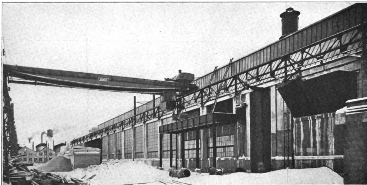
Fig. 6—The craneway serving the raw material storage yard, the centrally located concrete sand bins, the inclined hopper for sand going to the mixer and the extension of the charging floor platform for the receipt of pig iron and coke for the cupola
